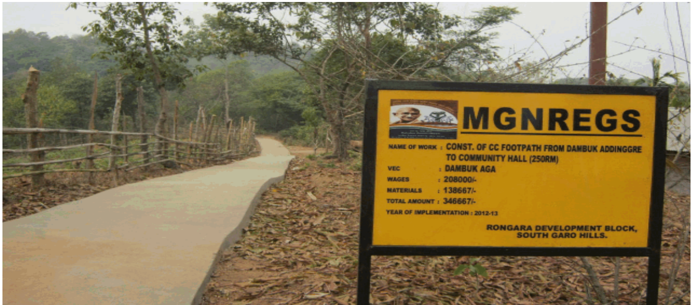
CONSTRUCTION OF CC FOOTPATH AT DAMBUK AGA VEC, RONGARA C&RD BLOCK, SOUTH GARO HILLS
