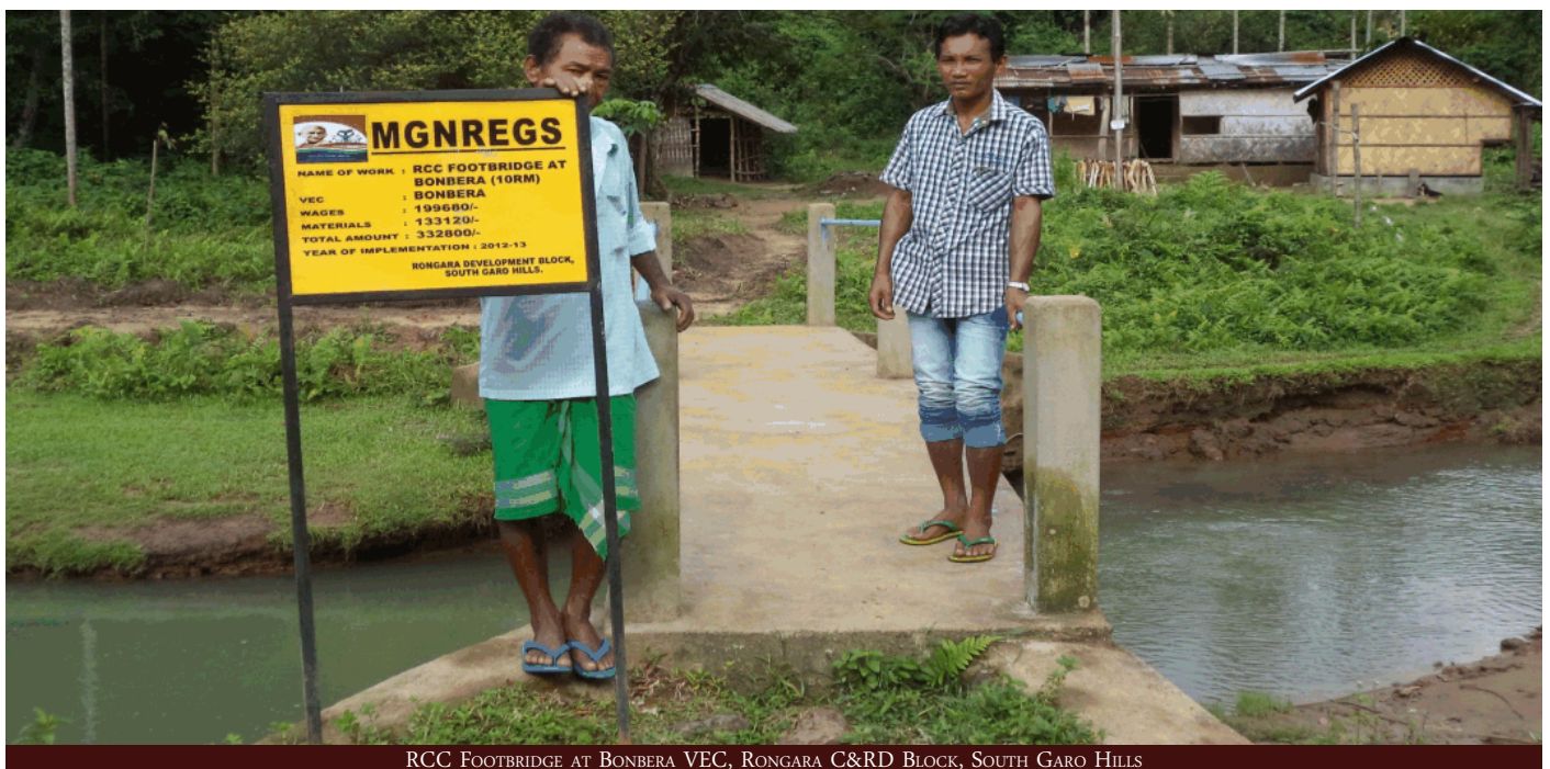
RCC FOOTBRIDGE AT BONBERA VEC, RONGARA C&RD BLOCK, SOUTH GARO HILLS
