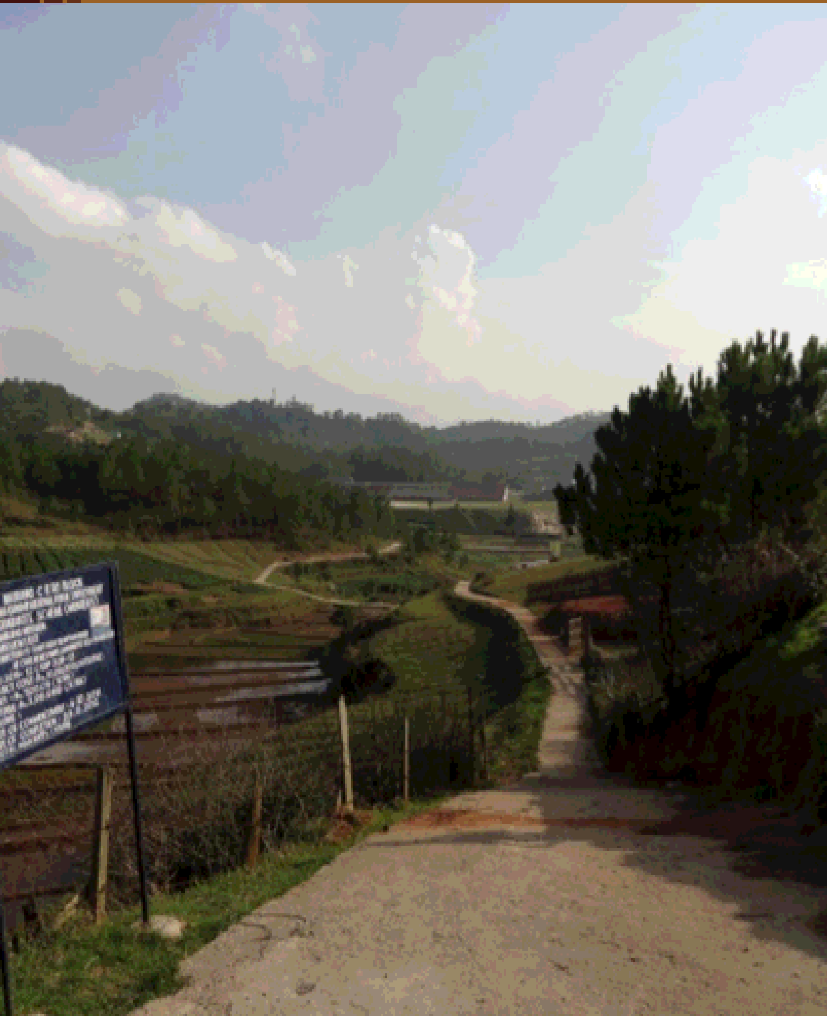
CONSTRUCTION OF C/C FOOTPATH FROM PWD ROAD TO KSA PLAGROUND, MAIRANG MISSION AEC, MAIRANG BLOCK, WEST KHASI HILLS DISTRICT
