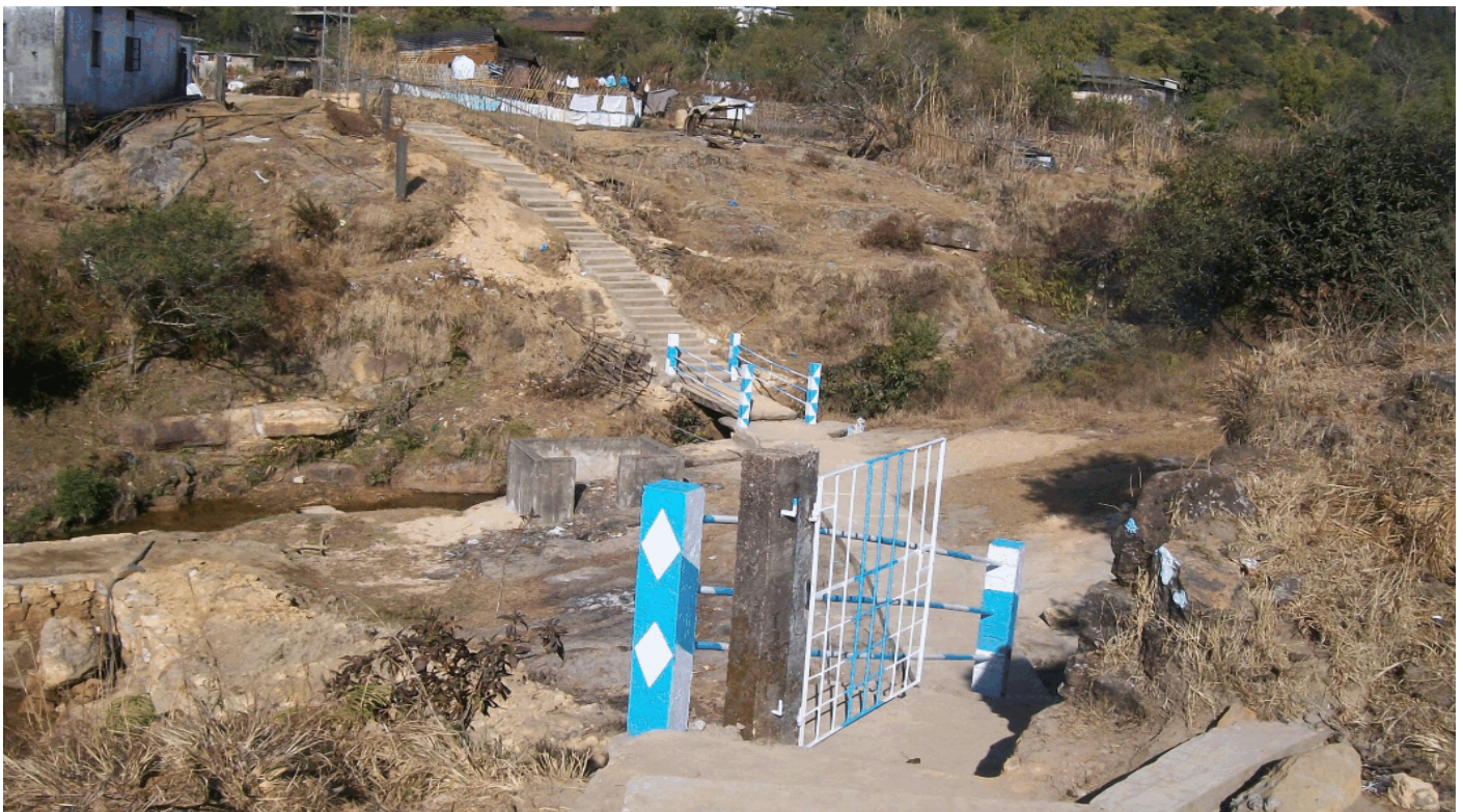
FOOTPATH AT LAITMAWSIANG, KHATARSHNONG LAITKROH C&RD BLOCK, EAST KHASI HILLS (AFTER CONSTRUCTION)
