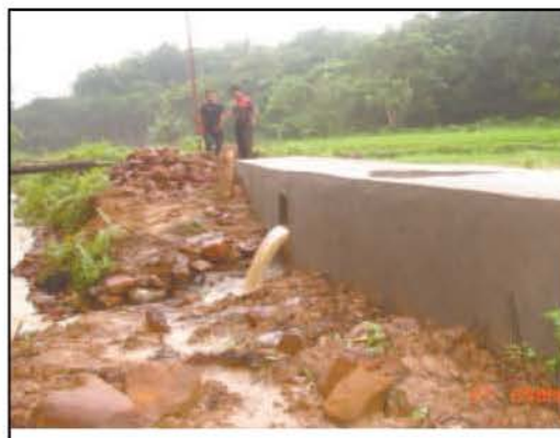
Earthen Dam with c.c core wall Ampanggre AEC, Rongara Block, South Garo Hills
